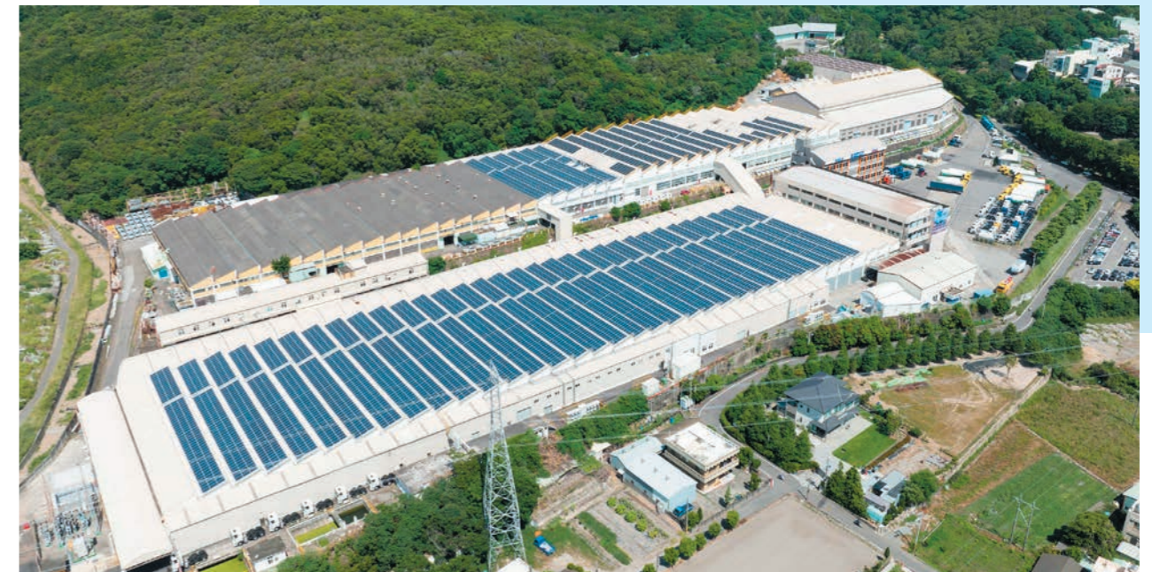
..... FPG vigorously plans to build solar power facilities
