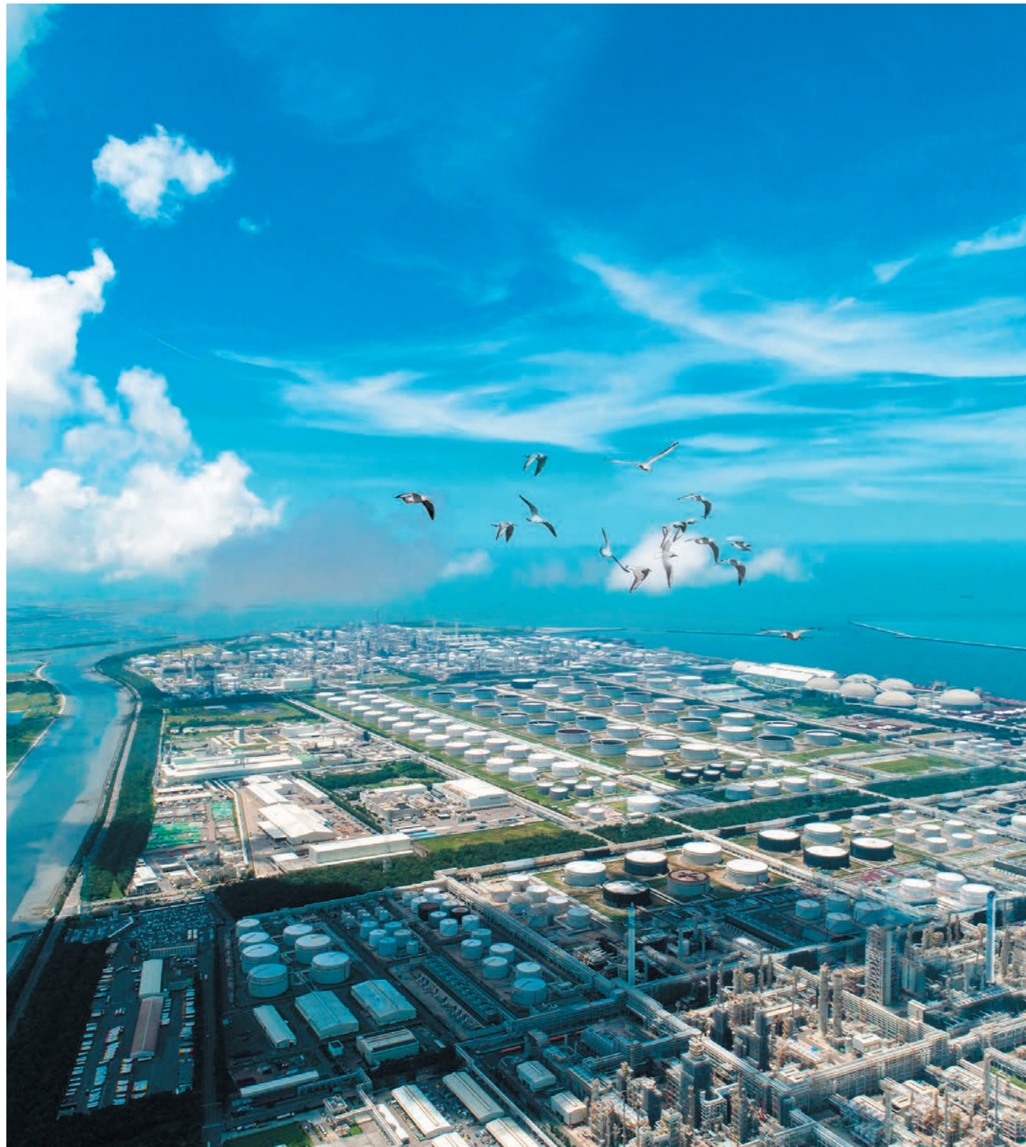
..... Mailiao Industrial Complex
